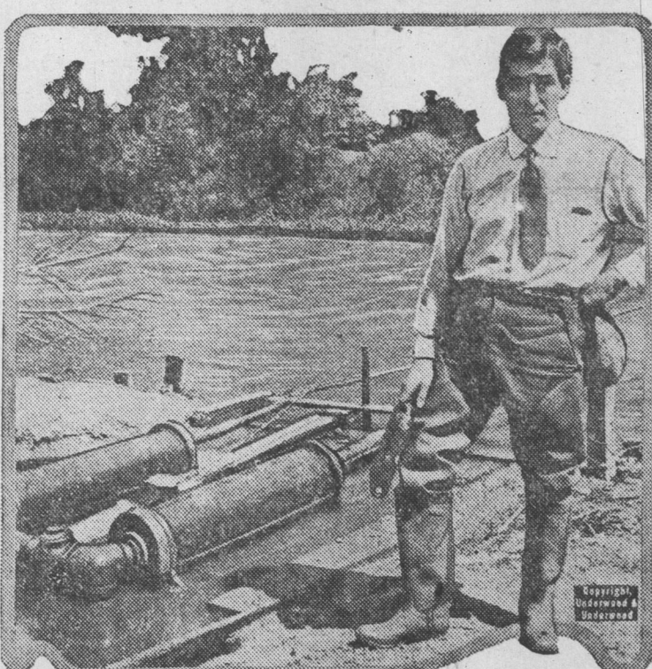
F. L. Gilman of Los Angeles, and his wonderful water pumping plant. This new motor, anchored in midstream sways back and forth, operating the two pistons shown in the photograph. It pumps 80 gallons of water a minute, and will make it possible to irrigate thousands of acres of land now arid.
