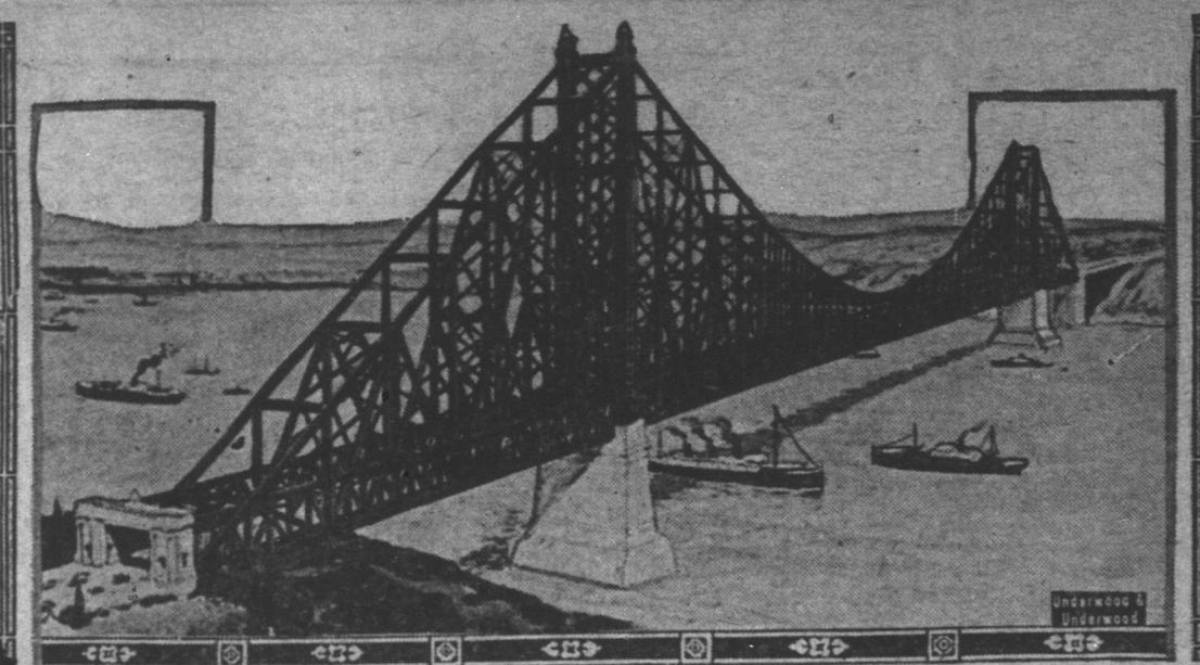
Artist's drawing from latest plans for the Golden Gate bridge at San Francisco, Cal., plans for which have just been approved by the United States War department. The cost of the giant structure, which is to stretch from Lime Point, at the Presidio, to the Marin shore, is estimated at \$21,000,000. The bridge will be of a new type of cantilever construction, its main span being 4,000 feet, or more than double that of any other span's length, and it will be 210 feet above the water.
