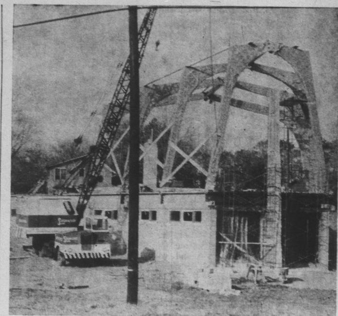
HUGE BEAMS — These huge laminated beams were recently installed on the St. Martin De Parres Catholic church near Lake Wawasee. Father Eugene Zimmerman reports the beams were a "long time coming from the west coast." The building project was started last summer. A Mail-Journal staff photo.
