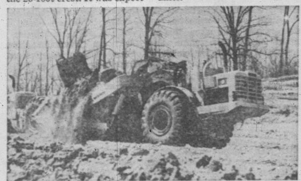
Machines beat the river. A fleet of giant Allis-Chalmers earthmovers worked around the clock against the rising waters of the Mississippi river near Muscatine. They poured in tons of dirt to build a levee (right) protecting farm land, industry and homes. The job was finished just hours before the river crested.
