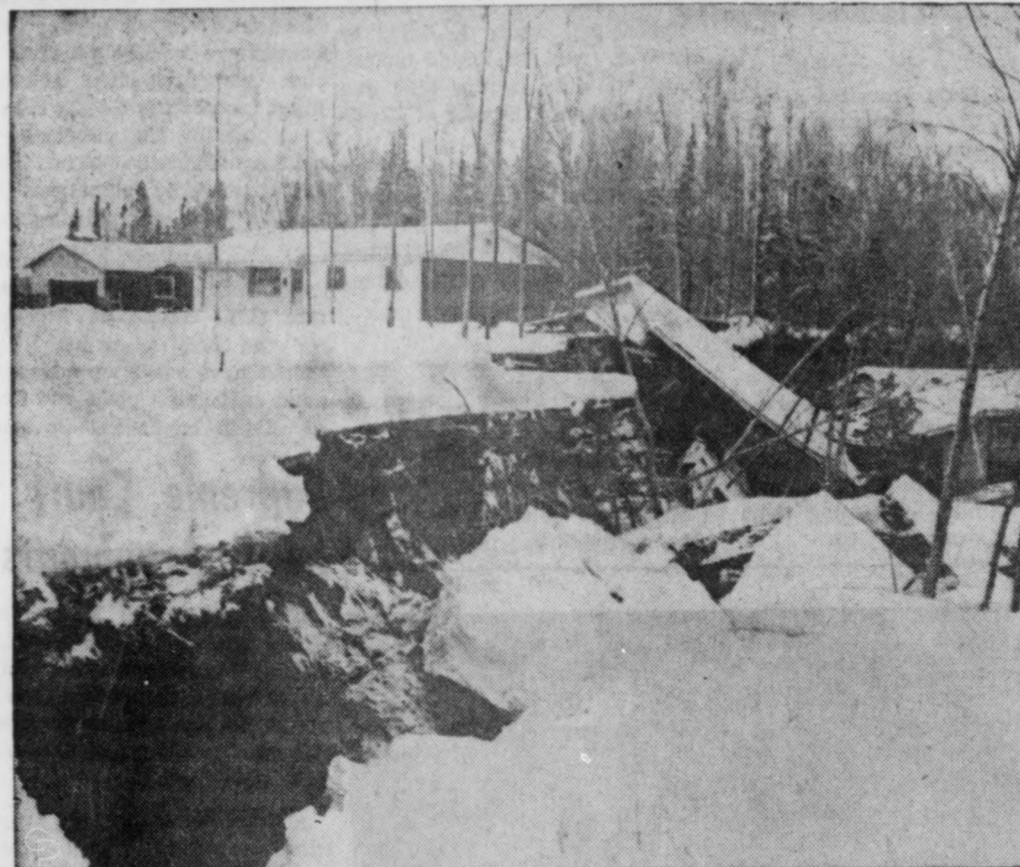
THE FAULT LINE opened by the earthquake in this Anchorage residential section separates this neighborhood in two, with the houses on the right dropped more than 30 feet.
