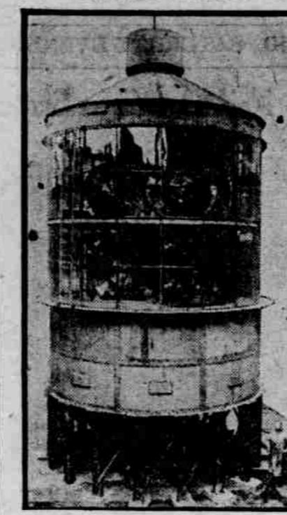
Regarded as the most powerful instrument of its kind in the world, this billion-candlepower scintillator guides airplanes on journeys to and from France. It has been erected at Dijon, France. The illumination comes from powerful electric arcs, convertible, where current is not available, to acetylene gas or paraffin vapor. It revolves to give flashes at regular intervals. Compare the size of the beacons with the man at the right.
