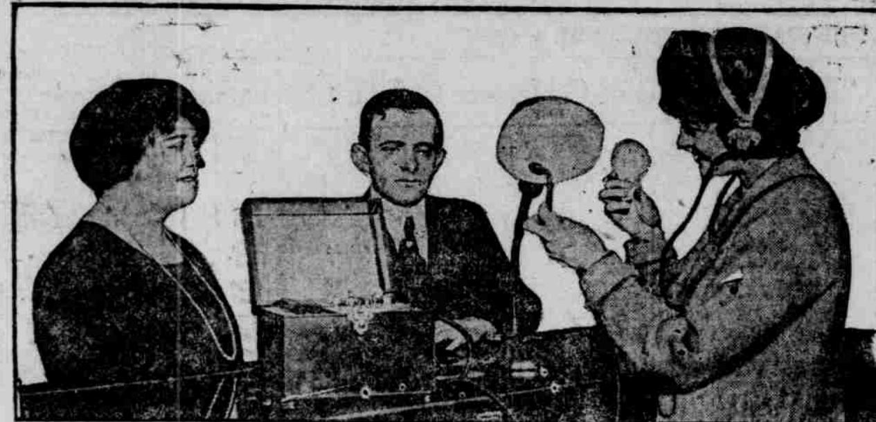
How to get radio music or message by just using an electric light socket is being demonstrated above by Miss Alice Slevin, of the Manhattan Supply Company. This method, invented by Major Gen. Squier, U. S. A., chief signal officer, does away with the usual receiving antennae. He conceived the idea less than week ago.
