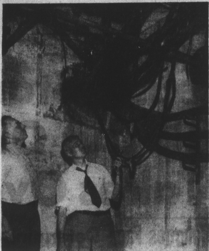
SEARED CABLES—Anderson utility officials Frank C. Yarling and Arthur Hoesek check flame-stripped cables that caused rupture in city-owned municipal power plant yesterday.
