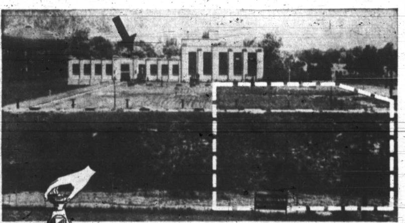
Additional purification facilities at the Fall Creek Station include a duplicate pretreatment basin (foreground, within dotted line), which, with six new filter units installed in the rear of the filter building (arrow), increased the daily production capacity from 15,000,000 to 32,000,000 gallons of safe water.
