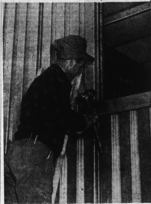
The aluminum industry has been busy with new products, one of which is quickly assembled, fibre-glass filled siding and sills. Here Emil Kalwat, 6038 Guilford Ave., is putting sill siding on the new Home-Made Pie Co. building.
