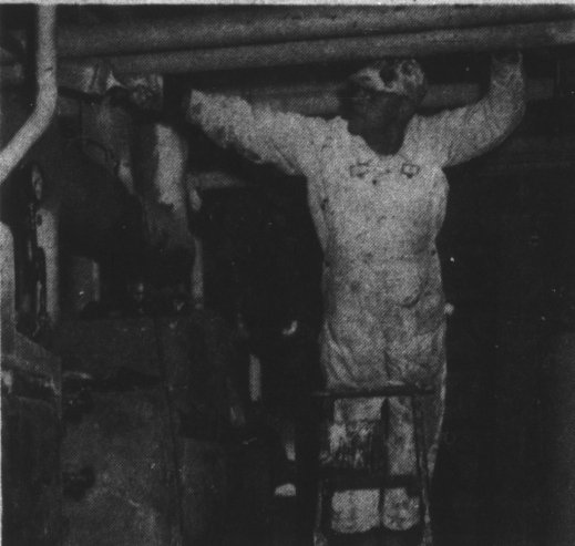
REPAIRS—Children at Lowell School are being inconvenienced while repairs to the building are being made. Here a workman paints pipes of a new boiler installed this year. New equipment takes the school's water system.
