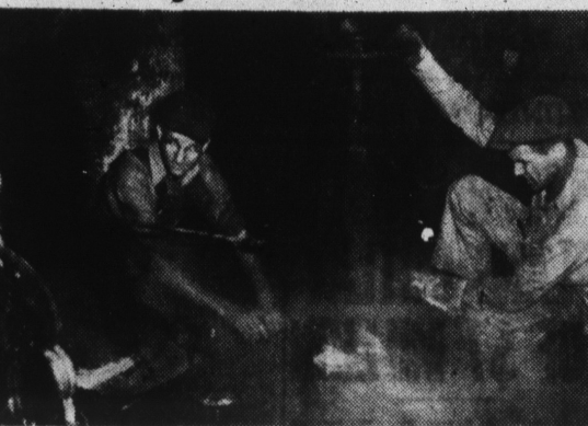
When a big turbine caught fire this morning at the Indianapolis Power & Light Co. plant, 336 Kentucky ave., firemen and employees worked furiously for half an hour to extinguish the flames. Shutting off oil to a pipe which burst and sprayed oil over red hot steam lines, causing the fire, are (left to right) Spencer Cooper, machine shop foreman, and Austin Fyffe, acting assistant chief engineer.
