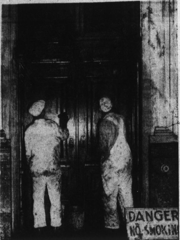
Painters resume work on woodwork in the state house after a flash fire in this doorway when a spark from a light switch ignited paint remover vapor. Quick-thinking painters extinguished the blaze before firemen arrived.
