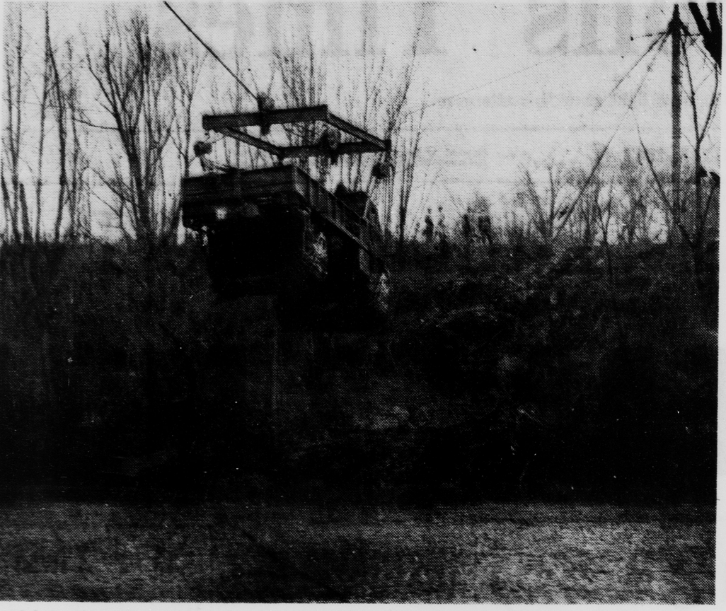
A heavy Army truck takes to the air as Armored Force Engineers at Ft. Knox, Ky., test a newly developed suspension cable bridge designed for transporting vehicles across small streams or gorges. The supporting column at right is made in knock-down sections, which can be floated. Tractors pull the vehicles across the stream by means of attached cables. The rig is said to be capable of carrying a light tank.
