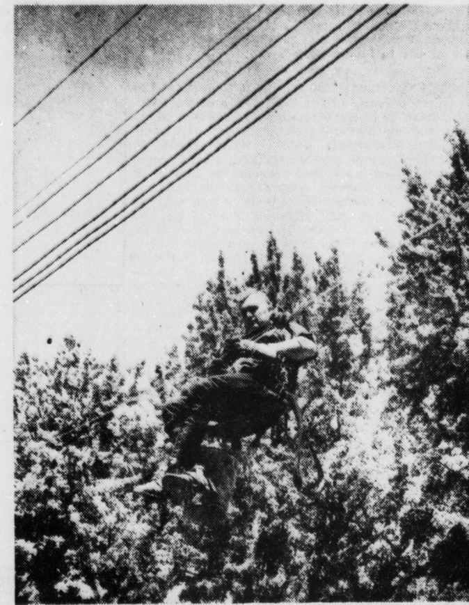
Willard Gardner, Indianapolis, is one of a telephone crew installing a 100-pair cable back of the high school for the notification ceremonies.
