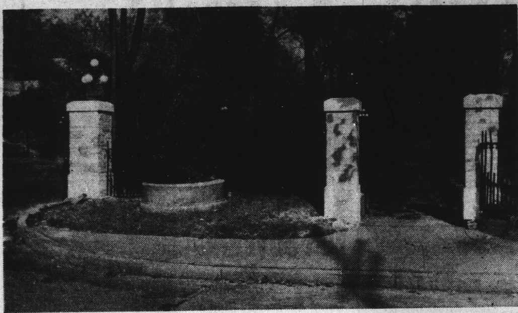
The 80-year-old iron posts at the entrances to Woodruff Place are being replaced by Indiana limestone portals. About a dozen new posts will be installed and will look like these at the corner of East Drive and Michigan St. Murray Morris, Board of Trustees member, said the old posts were rotting away inside and had become "dangerous."
