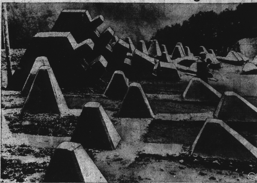
These mighty slabs of steel and concrete have all the appearance of ruins left by some vanished historic race. Actually they are tank barriers along the Siegfried Line by which Germany hopes to hold French tanks in check if war comes.
