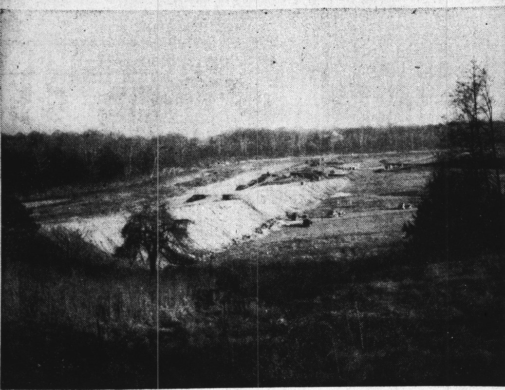
About 1000 men will work for nearly two years to complete the flood control program now under way from Cold Springs Road to 30th St. along White River. A general view of the Cold Springs Road end shows the levee, which will be topped with a boulevard, skirting the river and in the deep background can be seen the fill that will be the extension of 38th St.
