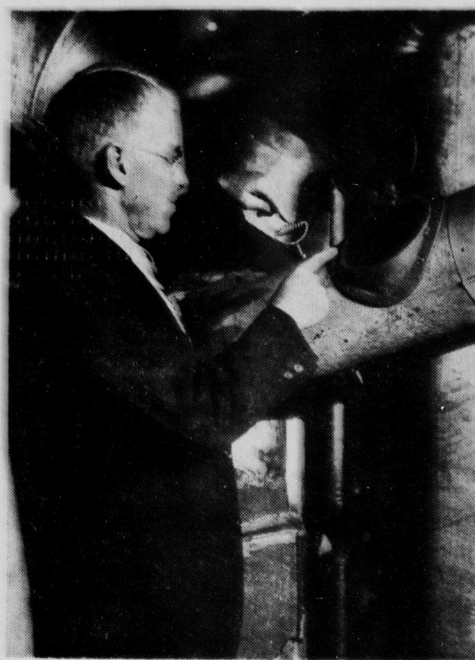
One of the positions for the check draft after firing is shown above. With his left hand, the demonstrator points to the butterfly damper, which should be between the check draft and the smoke outlet.
