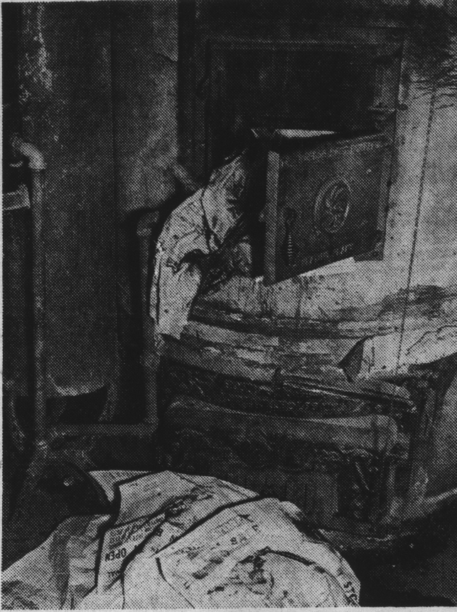
The furnace is a safe heater, but when papers are allowed to accumulate around its base, then it becomes a real hazard. Firemen report that they daily find this condition in basements.
