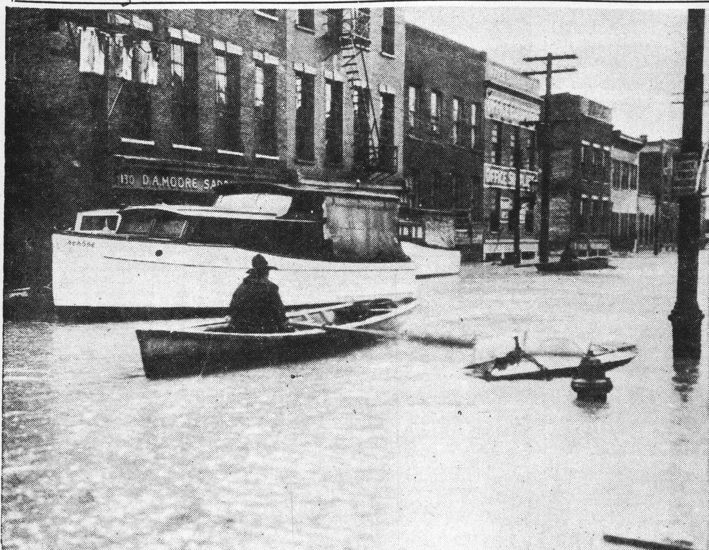
Downtown Louisville stores are flooded.
