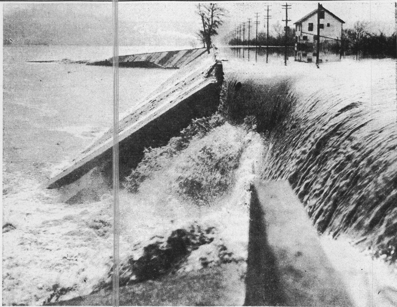
The Ohio pours through a gap in a Cincinnati levee.
