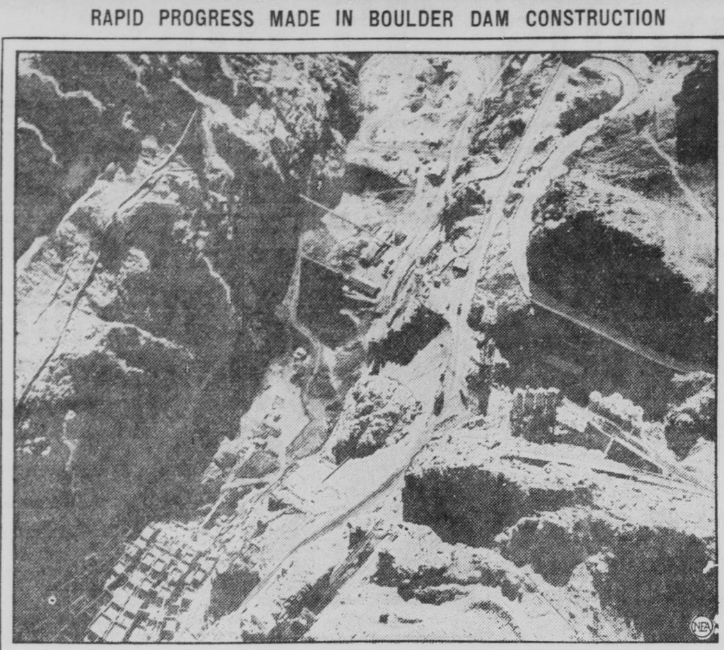
Progress of work at Boulder Dam is shown strikingly here, in an aerial view taken downstream from the dam, picturing the dry bed of the Colorado river gorge, where the water has been diverted, the dizzy winding road that leads to the works, and the concrete forms of the gigantic dam at the lower left.
