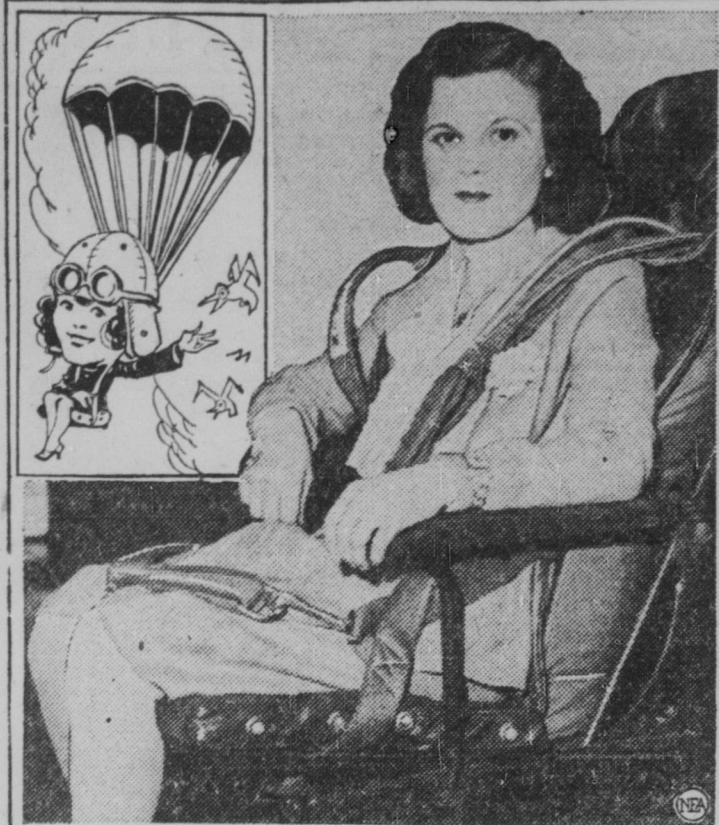
It's as easy as falling off a log" to use this nifty new "armchair parachute" for passengers in cabin airplanes. The chute is attached to the seat and all the wearer needs to do is jump from the plane when danger threatens and float to earth in a sitting posture, at least, that's the theory. Josephine Forbes is shown above as she demonstrated the new device at the National Aircraft show at Detroit.
