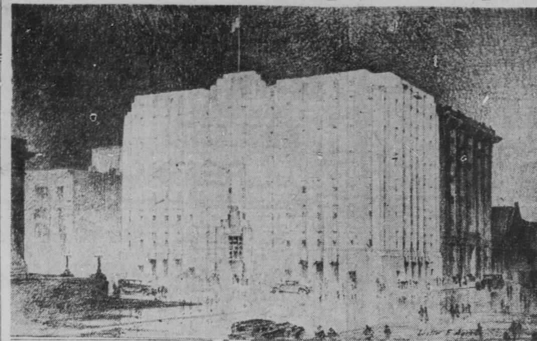
J. F. Carroll of the phone company. It is to be completed in 1932. Constructed of structural steel and reinforced concrete with an exterior facing of Indiana limestone, the phone building will harmonize architecturally with other new buildings surrounding the Memorial Plaza north of the business section.
