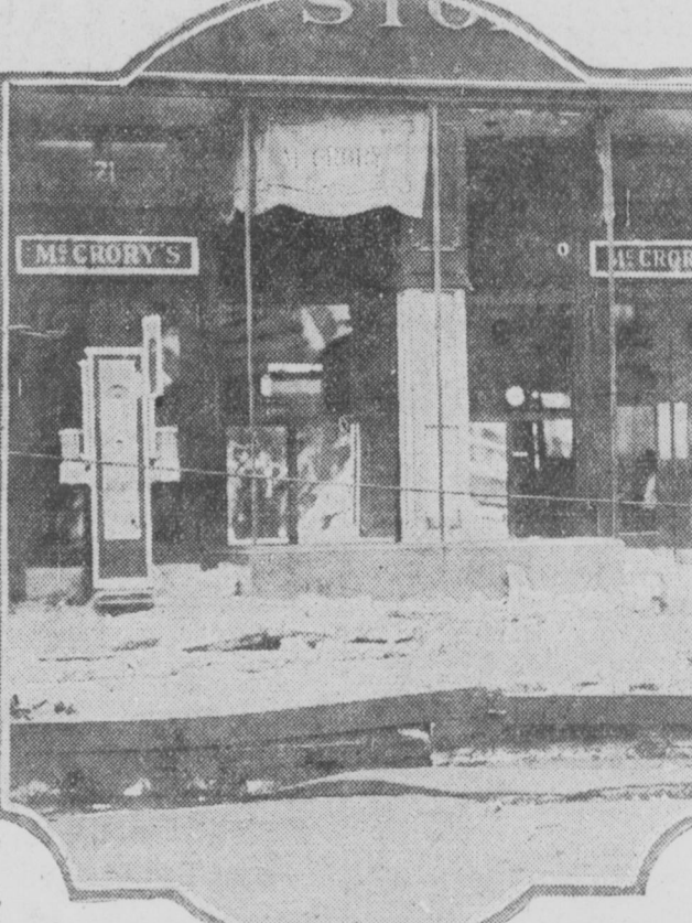
This picture shows damage done by the explosion in the basement of the McCrory's 5 and 10-cent store, 19 E. Washington St., early Sunday. The blast is believed to have been caused by sewer gas.
