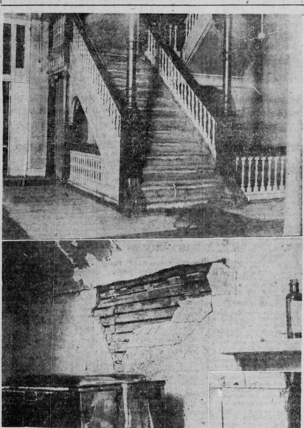
Scenes in the old city hospital building, which has been branded a fire-trap by inspectors. Above—The main, all-wood stairway. Below—A broken wall in the sterilizing room. Inset—A rat hole, stopped with tin, in the rear hall of the first floor.
