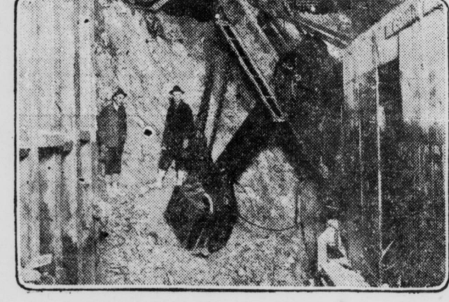
Above is a diagram showing how the railroad tunnel and the parallel water tunnel pierce the heart of the continental divide. Below is a steam shovel removing crumbled shale and rock after a blast had been let off in the tunnel shaft.
