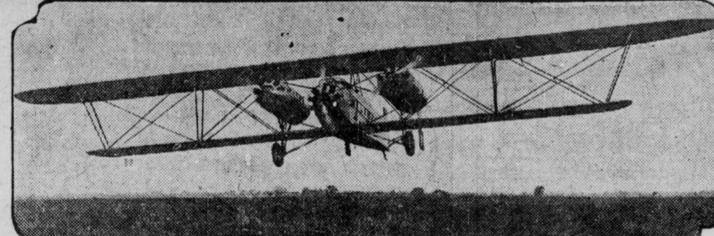
The great triple-motored Sikorsky plane in which Capt. Rene Fonck and his companions plan to make their non-stop flight from New York to Paris here is shown in test flight at Roosevelt Field, L. I. The wings have a spread of 150 feet across, and the plane will carry 25,000 pounds.
