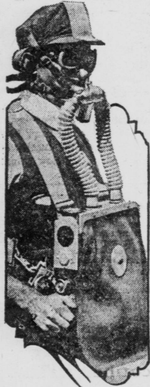
John Landau of the Brooklyn navy yard experiments with a breathing apparatus recently perfected by the bureau of mines. An oxygen tank permits the wearer to stay under water fifteen minutes and to pass through thick smoke.
