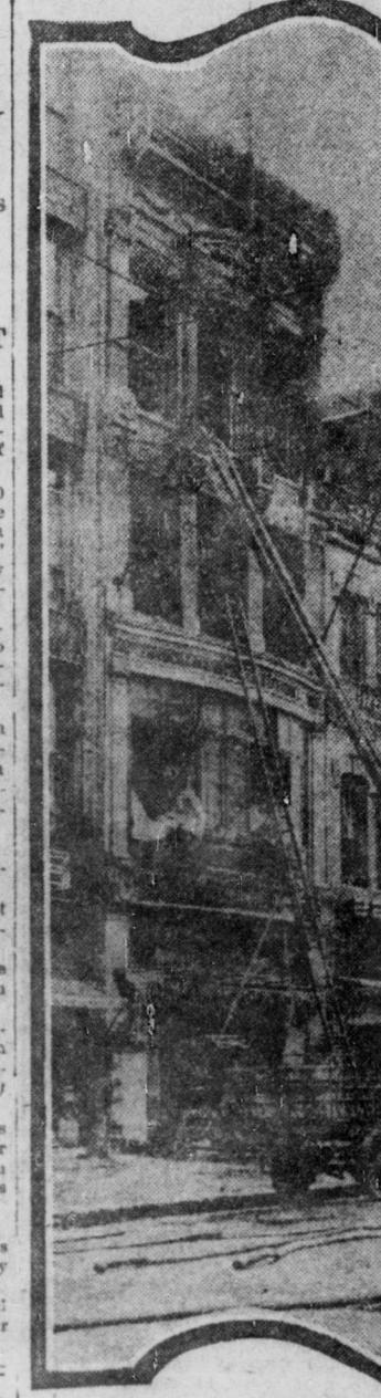
The completeness of the destruction of the store of the H. Lieber Company is shown by the above picture of the empty shell of the structure. The fire in its early stages blazed so fiercely that firemen were compelled to leave the ladders and depend on a water tower. Adjoining buildings were saved by heavy fire walls.
