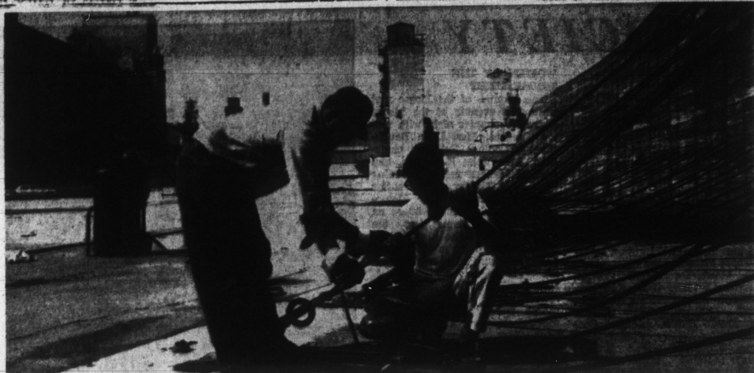
TIGHTENING UP — Central Soya's Decatur plant is in the midst of its annual preparation for the coming soybean harvest. Above Bob Morris and Gary Covert adjust the cables on the plant's large bean storage "bowl." —(Photo by Cole)
