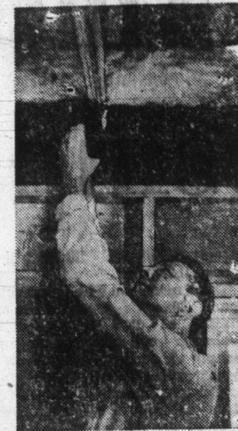
INSULATION HELPS convert unfinished attic for comfortable living. Mineral wool batts are stapled in place with vapor barrier facing heated area.
