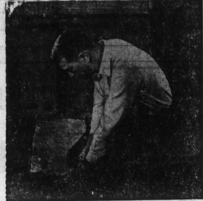
BATTS OR BLANKETS OF INSULATING material can be cut easily with knife or scissors when odd-size pieces are needed — important, since to achieve best results while insulating an area, all irregular crevices should be filled. In use here, mineral wool.
