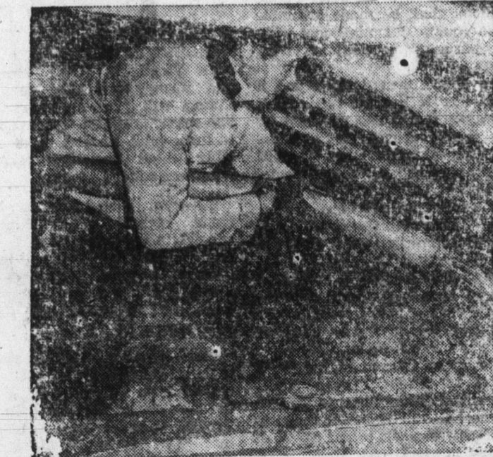
DO-IT-YOURSELF FANS SHOULD CALL IN professional help, when "blowing wool" insulation is used. Here, insulation mechanic is shown filling spaces between attic joists, with the use of a pneumatic hose brought in through ventilation opening.
