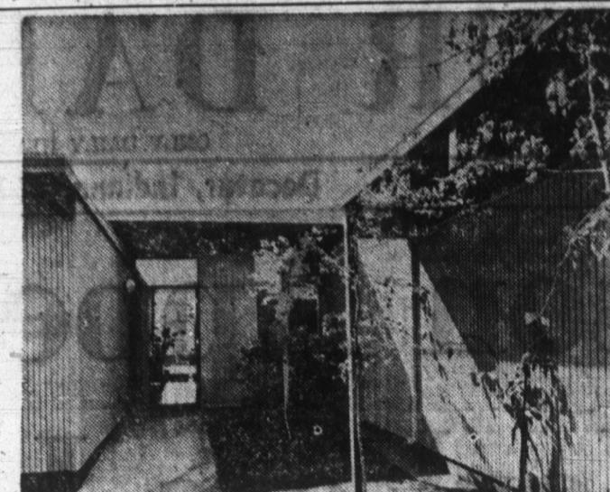
This is the attractive exterior of a home with sheathing and siding combined in one  $\frac{1}{8}$ -inch thick fir plywood panel. Texture One-Eleven, a vertically-grooved material popular all over the country, was used here. The strength of this wall resists shocks of earthquakes and high winds better than conventional construction, and cost is about \$350 per house less than other methods.
