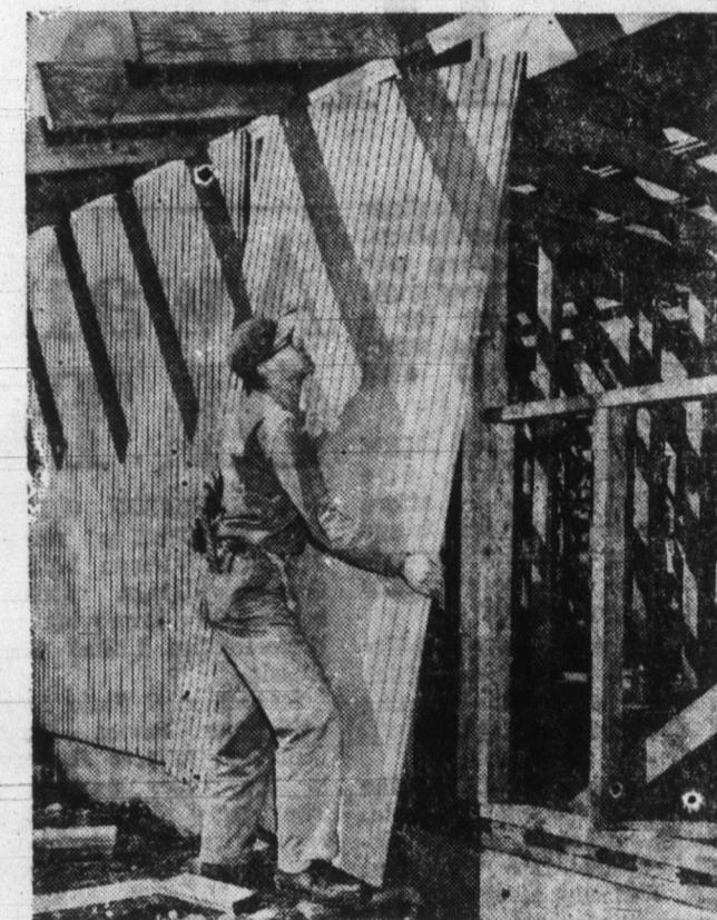
A panel of Texture One-Eleven goes quickly into place, provides an attractive finished siding as well as sheathing that serves also as wall-bracing. This fir plywood panel makes a wall twice as rigid and nearly three times as strong as one conventionally built. Builders all over the country are adopting this system.
