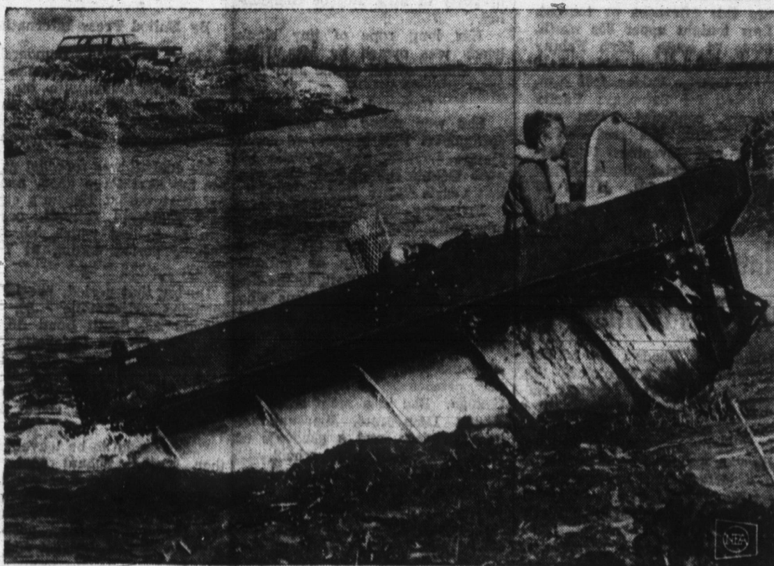
"OVER LAND, OVER SEA . . ."—When this new military vehicle runs aground, it keeps right on going. The craft rides on two rotary metal pontoons fitted with spiral blades that move it forward, backward and even sideways. The blades clean themselves as they dig into swampy bogs, snow or soft earth. Weighing about a ton, the craft, called the Marsh Screw Amphibian by designers at Chrysler Corp., reaches its top speed in deep snow, about 20 miles an hour. Speed in muck is about 10 miles an hour. It is shown during initial tests in the swamp and bayou country of Alabama and Louisiana.
