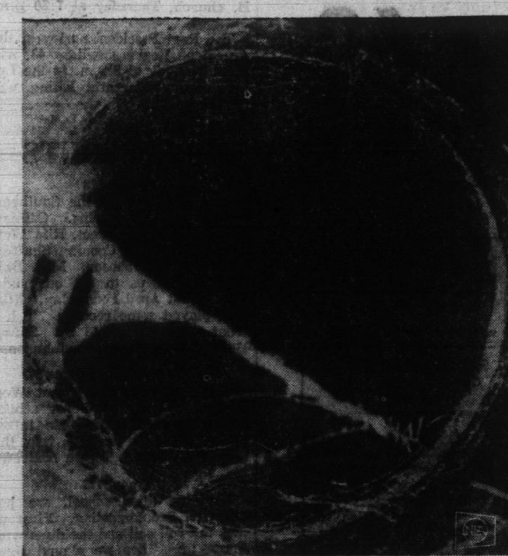
THE CULPRIT —Photo taken by drainage line camera reveals root that has entered between two tiles and bridged itself across the drain.
