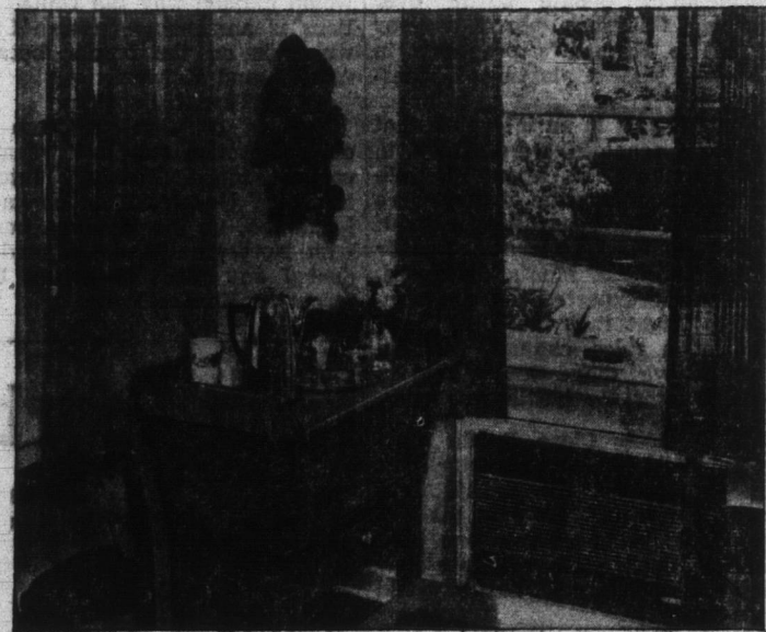
A through-the-wall electric room air conditioner installed in this new Gold Medallion Home leaves window with unimpaired view and gives freedom of decorative treatment. Like window units, wall air conditioners cool, dehumidify and filter air.
