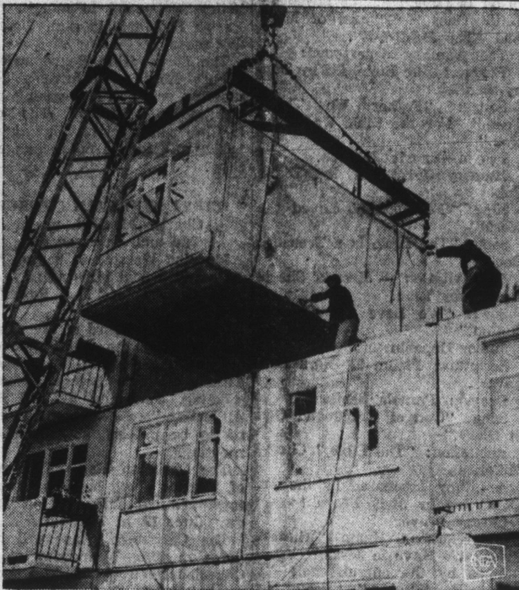
HOUSE OF BLOCKS—Workers guide a large, boxlike room into place during construction of a four-story apartment house in Krasnodar, U.S.S.R. The prefabricated concrete units containing doors, windows and plumbing facilities are being built to alleviate the country's housing problem, according to information from an official Soviet source.
