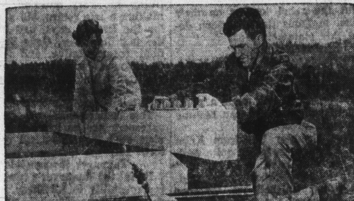
(Western Pine Association) CONCRETE BLOCKS serve as foundation for cabin. 4" x 10" joists are spaced 4' apart on 4" x 10" Fir or Larch beams.
