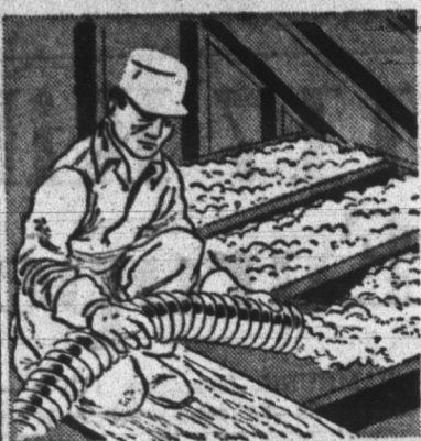
Floor of attic is insulated by workman using special pneumatic equipment developed by mineral wool engineers. Air pressure distributes the insulation evenly and thickly for most effective heat barrier.
