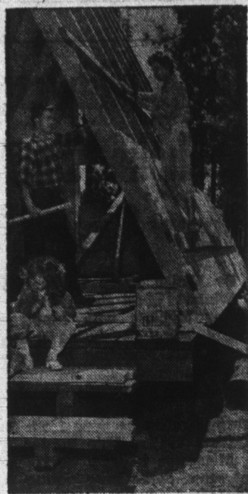
(Western Pine Association) SHEATHING of the all-in-one roof and side walls serves also as interior finish wall of cabin.
