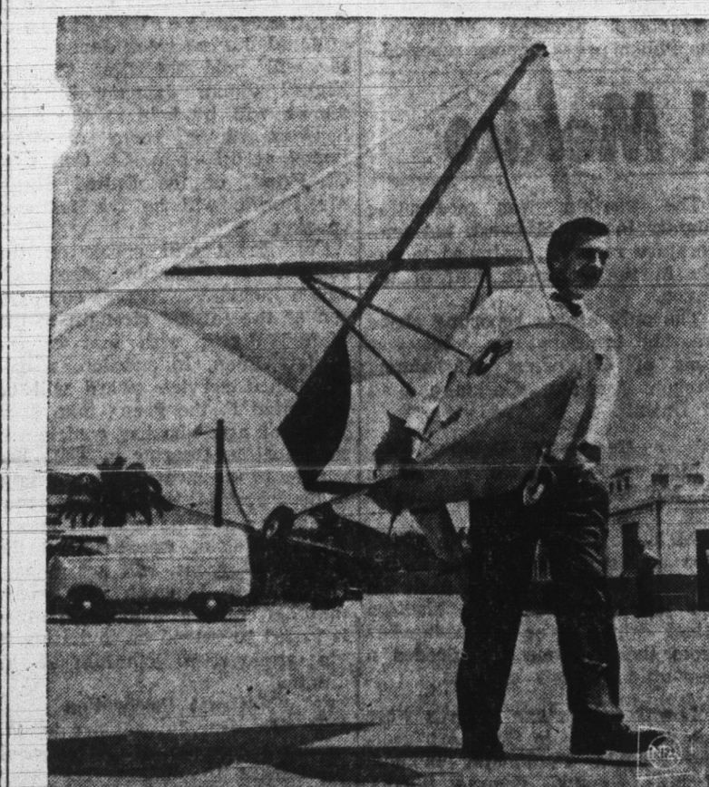
SAIL-PLANE —A small drone version of the experimental Flex Wing aircraft is being investigated by the U.S. Marine Corps at its desert facilities at Twenty-Nine Palms, Calif. The plane would be powered by a gasoline engine in the rear. Launched by troops in the field, it would serve as a reconnaissance or spy plane. Like its larger counterpart, the drone has a "wing" of fabric and is a light aircraft for Ryan Aeronautical Co. employee Cecil Craig to carry.
