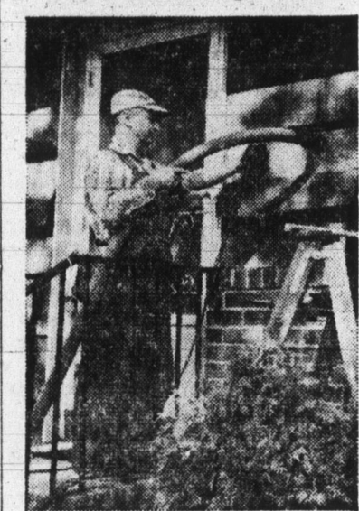
Workman uses air pressure to force loose mineral wool into every crack and crevice in wall of this home. When all outside walls, attic crawl space, and floors have been filled, a complete blanket of mineral wool will keep heat in during winter and out in summer. Homes will be sealed and siding replaced to look like new.
