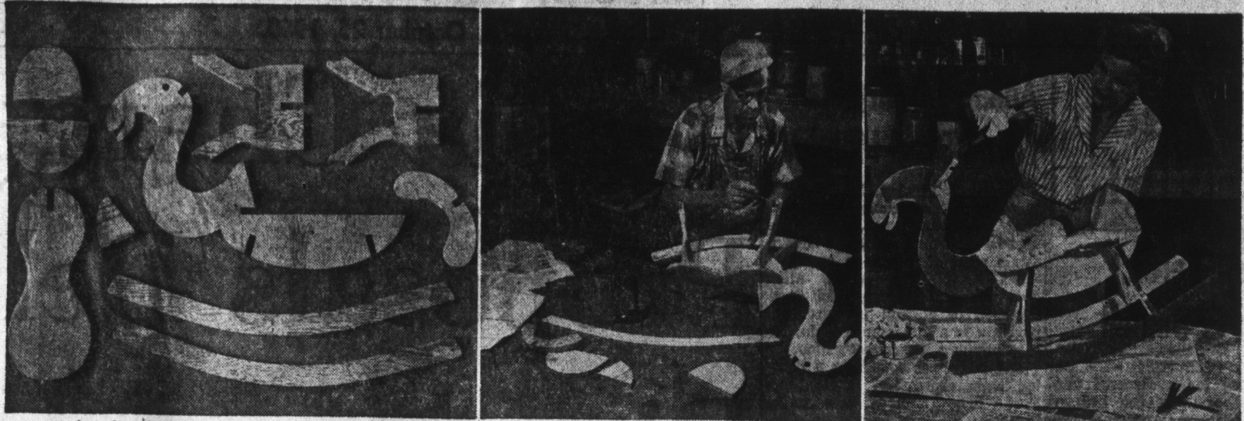
Here are the three simple steps for building a member of the Plywood Zoo. The pieces are cut from a 3x4-foot piece of 1/4-inch fir plywood (left), slipped together and fastened with glue and nails (center), and then painted.
