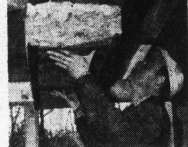
Workman lifts 6-inch batt of mineral wool insulation into place between ceiling joists of house being insulated for economical air conditioning.
