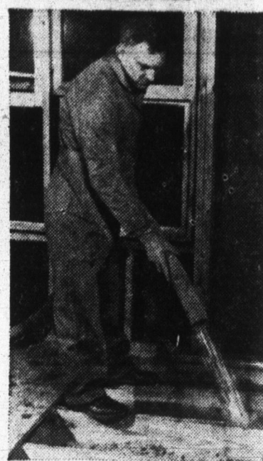
Workman installs mineral wool insulation in attic floor of an older home, using "blow in" system. This method, developed especially by mineral wool engineers to make insulating existing houses easier, employs air pressure to force the insulation into hard-to-reach wall spaces, floors, and ceilings.
