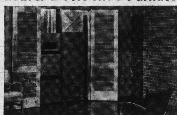
Ponderosa pine louver doors keep furnace and air conditioning unit from view in basement playroom, yet permit them to "breathe."
